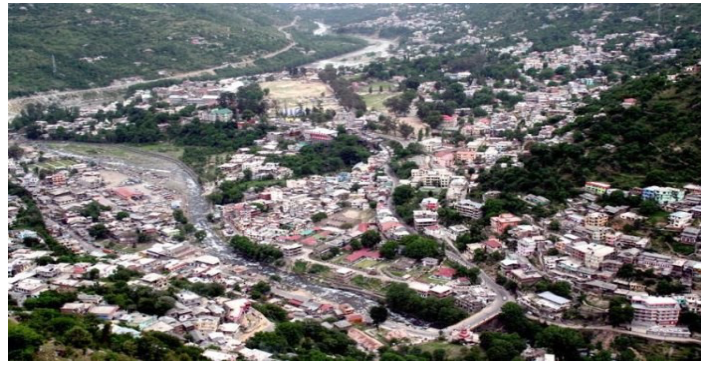
Haphazard Construction in Kullu Valley
