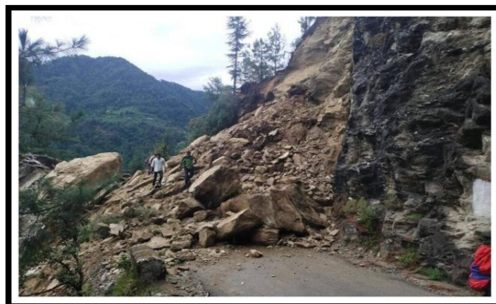
Image Showing Landslide
